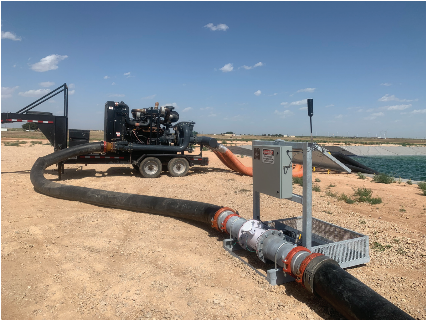
Pumping skid, with solar-powered controls.
